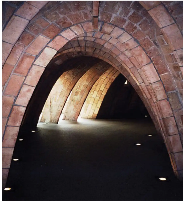
Fig. 4: Vault by Gaudí in the shape of a catenary arch.
