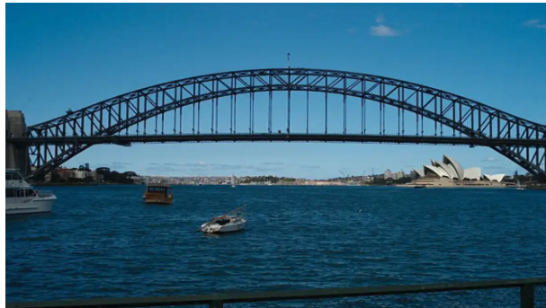
Fig. 2: Harbour Bridge in Sydney.
