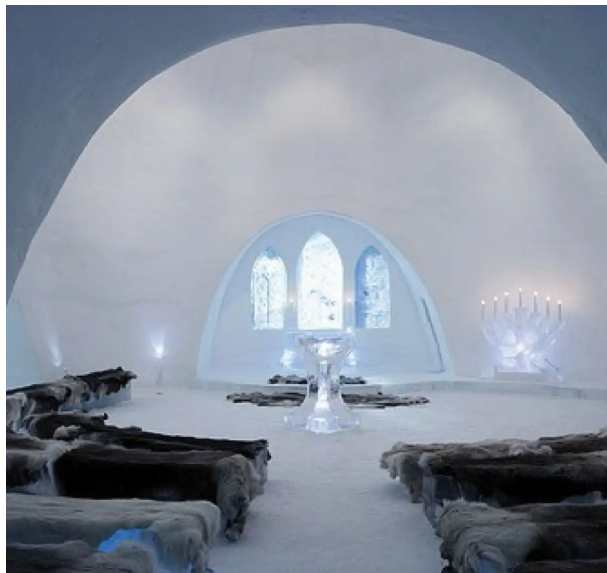
Fig. 5: Icehotel in Sweden in the shape of a catenary arch.
